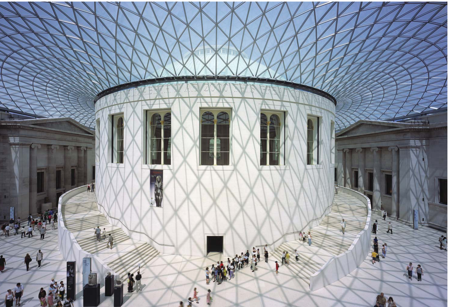
Figure 42: The court yard glass and steel gridshell after completion. The project was made in collaboration with Foster And Partners architects and Buro Happold engineers. Image source: [Williams, 2001]
