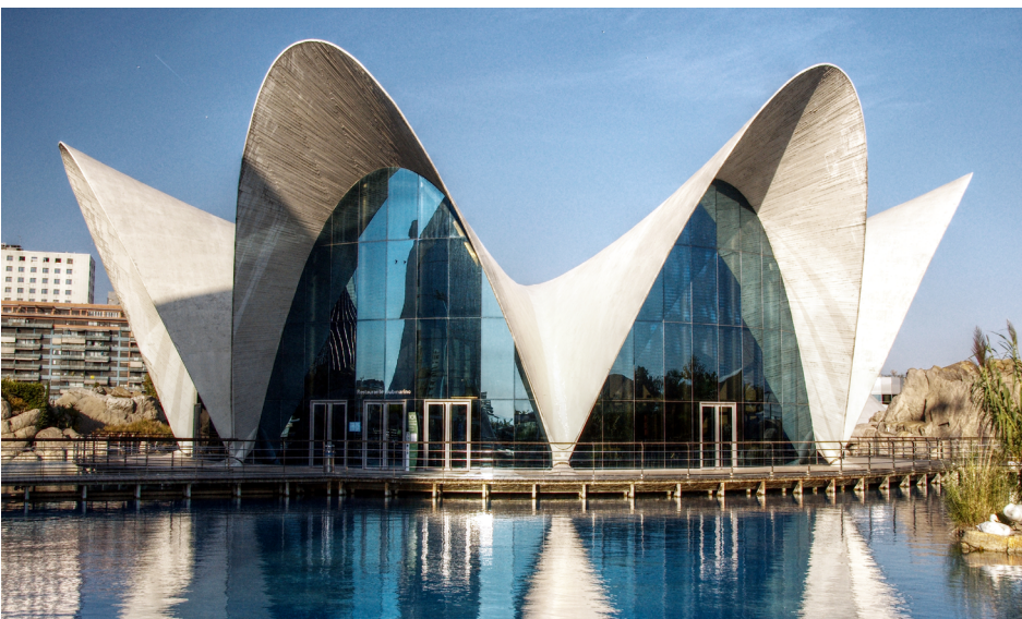
Figure 16: L'Oceanogràfic is a great example of structure that makes concrete appear lightweight when used as a shell. The design is a combined effort of the architect Félix Candela and engineers Alberto Domingo and Carlos Lázaro.
