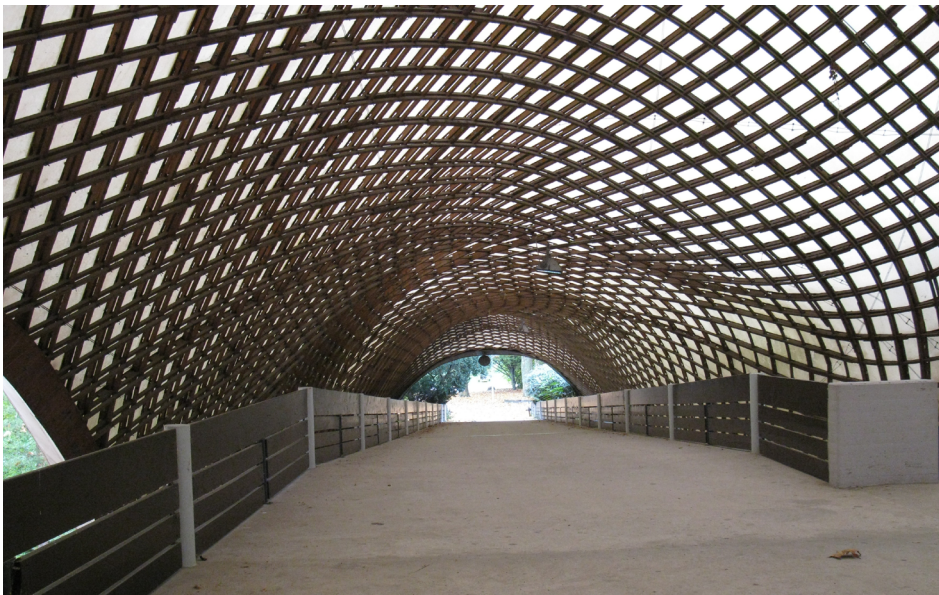
Figure 20: The Multihalle in Mannheim is considered a pioneering piece of architecture in terms of form finding. It was designed by Frei Otto in collaboration with Ove Arup & Partners structural engineers. The grid is build of a double-layered pinewood laths. The grid was build flat on the ground and then bent into its final shape by raising the grid and locking it in its supports. The shape of the grid was found using physical modelling. The physical model was a net of hanging chains to determine the structural geometry.
