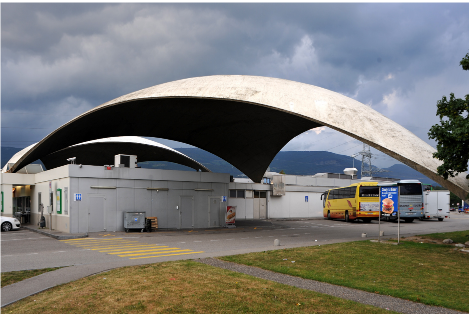
Figure 15: Heinz Isler (1926-2009) used physical modelling to find the shape of his magnificent concrete shells. This shell is a roof to a highway service area.
