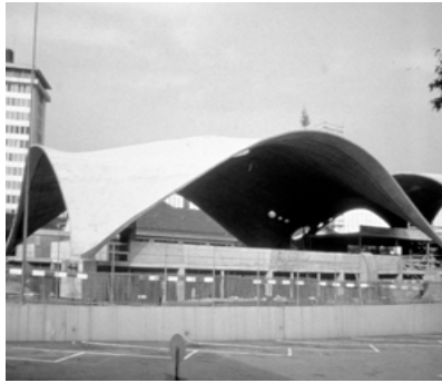
Figure 75: The roof for the Sicli company building in Geneva designed by Heinz Isler. The form is imitated using the dynamic relaxation component. Image source: http://www.ce.jhu.edu/
