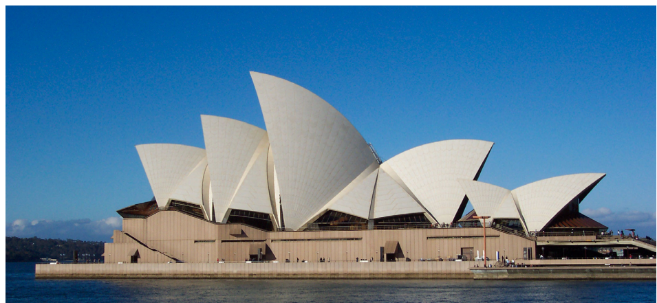
Figure 6: The Sidney Opera house is a brilliant example of magnificent structural design from a collaborative effort by the architect and engineer. Peter Rice is credited for solving the problematic geometry of the roof shells thus realizing the visions of the architect Jørn Utzon. Image source: http://en.wikipedia.org/wiki/File:Sydney_Opera_House_Sails.jpg
