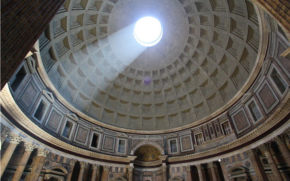
Figure 14: The most simple continuous shell structure is the semispherical dome. Throughout history these domes were erected using materials strong in compression such as bricks or un-reinforced concrete. Pantheon, build 126 AD, is made out of unreinforced concrete. Concrete, as a material was lost for ages. To this day, Pantheon is the largest un-reinforced concrete dome in the world. It spans 43.3 meters.
