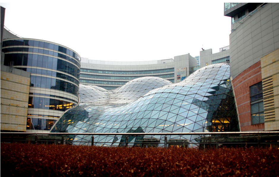
Figure 21: This curved free form gridshell structure is located in Warsaw, Poland and stood finished in 2007. It is designed by architects The Jerde Partnership International and engineered by Arup. The gridshell functions as roof covering a shopping area. The gridshell is composed of steel elements and triangular glass panels. The shape of the gridshell and the triangulaztion of the mesh was optimized using form finding which will be discussed in detail in chapter 3.4
